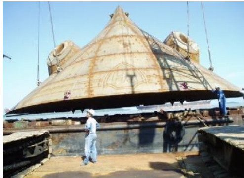
Fig. 3.3.2 Lifting Block for Loading
