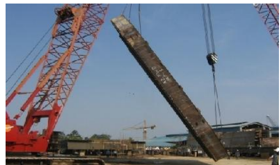
Fig. 3.3.1 Block's Overturning Lift
