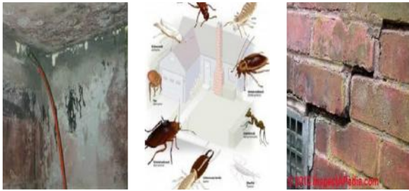
Leakage of Pest Poor
